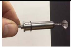
4. Use a small block of wood and a mallet to tap the cable at the point the cable is coming out of post to set the cable angle.
