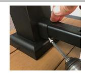
9. Apply adhesive tab (J) to flat surface of Top Rail (A) near the post. Slide Bracket Cover (D) to interlock with the flange on the saddle bracket.
