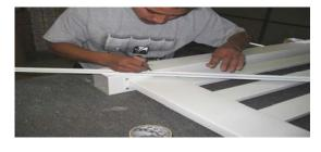
Attach the brace using 2 self-taping screws at each end of the gate as shown to the right. The screws are provided. Note: Marke the hinge side of sock post with tape. This will keep you from installing the angle brace in the wrong direction.
