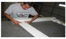
Once the gate is assembled, measure the width at the top and bottom of gate as shown here. They must be the same width or your gate will be out of square!
