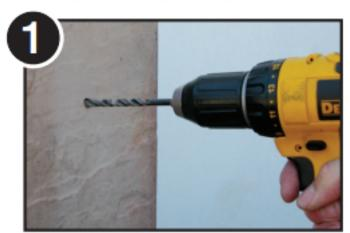
Drill 1/4" hole with masonry bit to 1-1/2" (minimum) depth.
