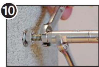
Tighten the lock-nut against the swivel component to prevent the fitting from loosening.
