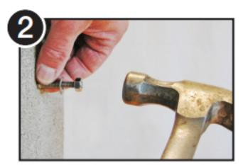
Carefully tap the Expansion Anchor (with washer and anchor nut).
