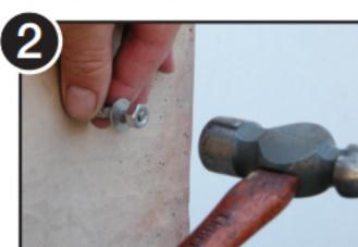
Carefully tap the Expansion Bolt until the machine threads protrude 3/4".
